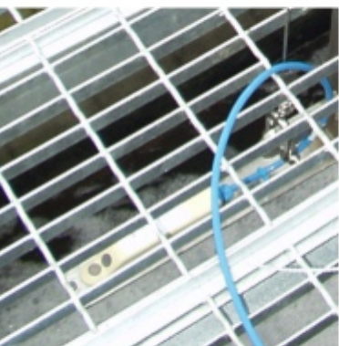
Lift-up mechanism for inspection purposes or for sensor removal under operational conditions
