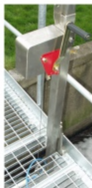
Lift-up mechanism for inspection purposes or for sensor removal under operational conditions
