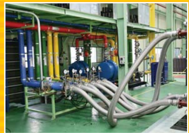
■ Pilot Testing Room
